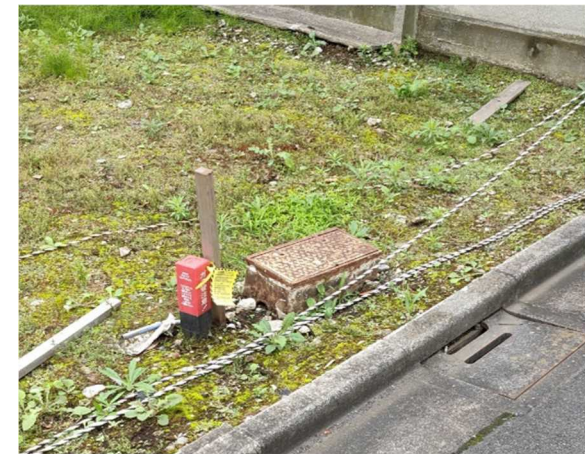
Fig.16 Service pipes not expected to be used
