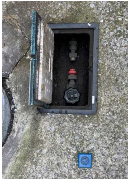
Fig.15 The service pipe where water meter has been disconnected
