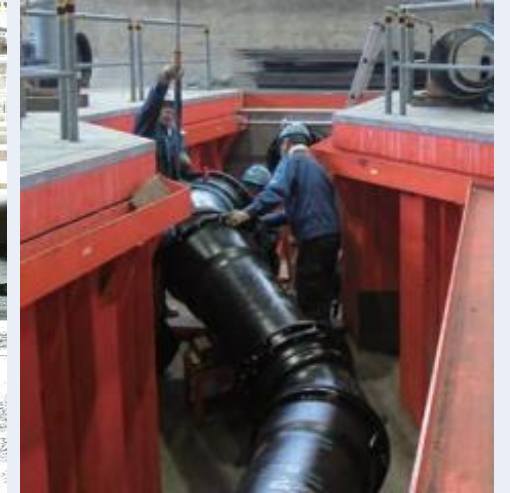
▲ Training to connect water pipes
