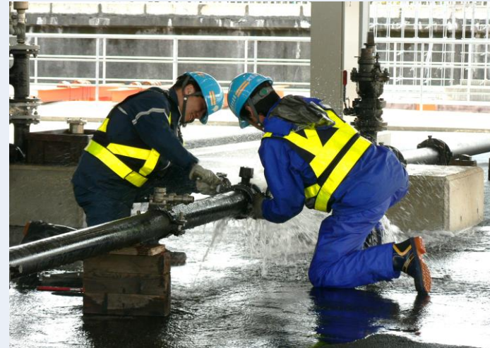
▲ Training to repair leaking water pipes
