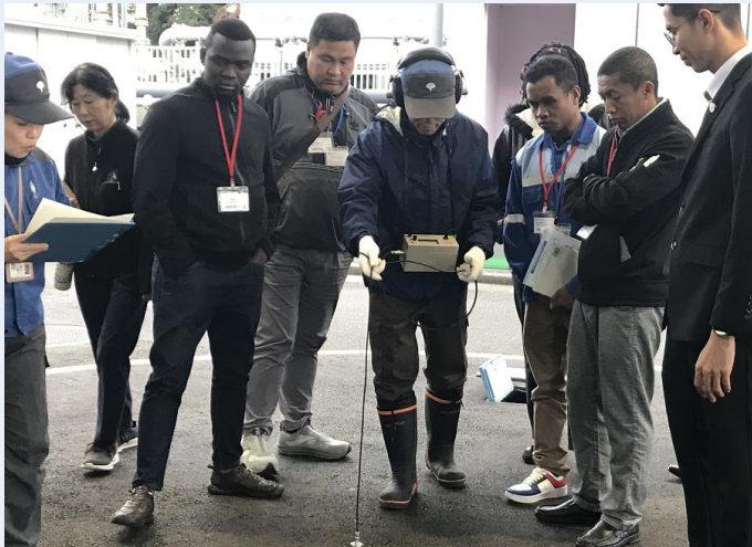
▲Drill for water leakage investigation
