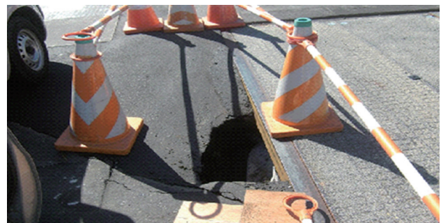
Road subsidence caused by heavy rain
