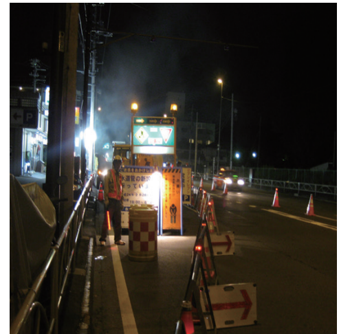
Work area safety facilities
