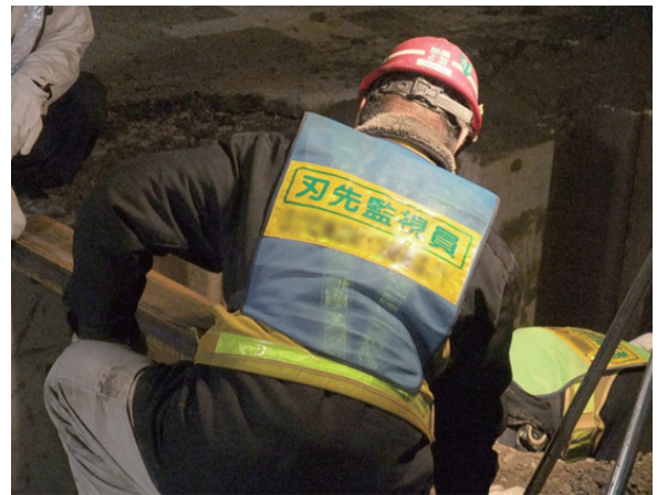
Advance hand excavation spotter
