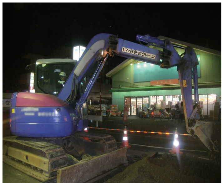
Backhoe with a crane function
