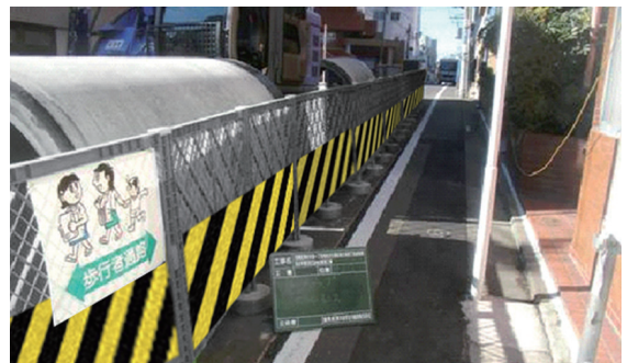
Separating walkways with plastic fences
