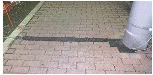
Cables are buried underground
