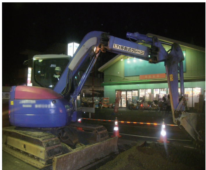
Backhoe na may crane function
