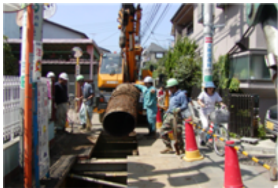
Photo 2: Replacement of aged pipeline
