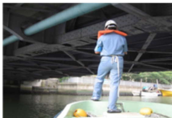
Photo 1: Diagnosis of pipeline attached to bridge
