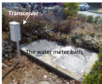
Figure 9 Transceiver installation (Facilities A and B)
