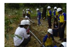
【Figure 7】 Scene with polyethylene pipe laying
