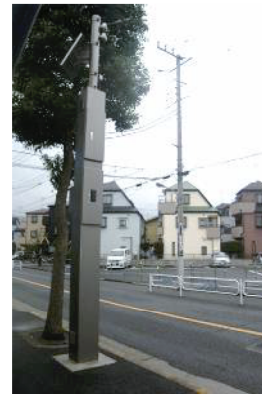
Figure 8 - Telemeter with combined casing/lead-in pole
