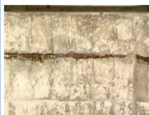
Exposed rebar on ceiling beams
