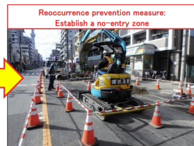
Figure 3: Accident case study and reoccurrence prevention measure for a frequently-occurring disaster: "Disaster caused by movement of dump trucks or other heavy equipment"
