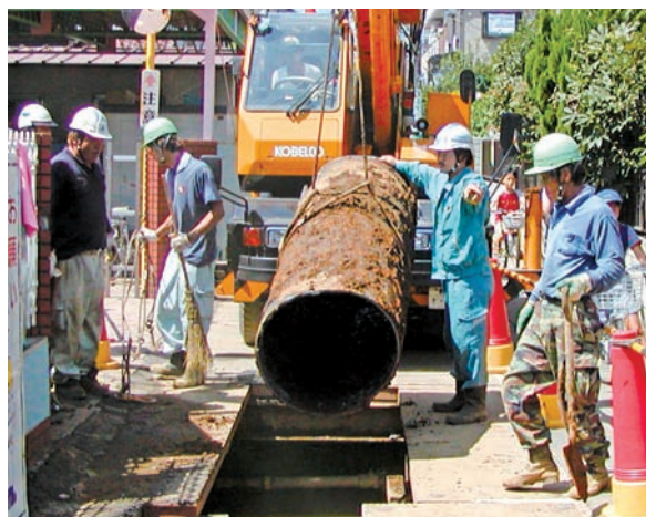
▲経年管の取替
