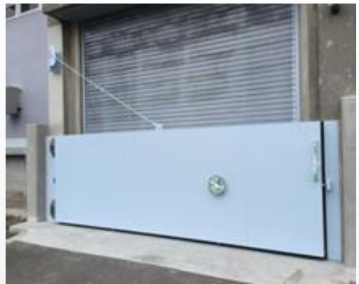
Installation of watertight doors
