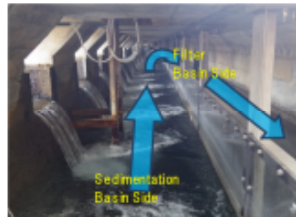
Figure 16 Partition wall and detour flow wall installed Figure 17 Partition wall installed in sedimentation water channel
