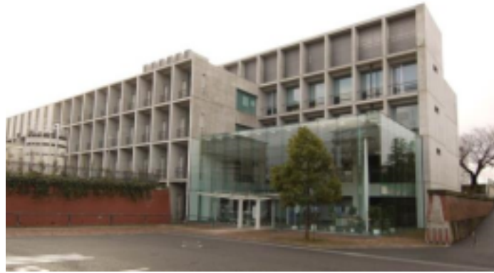
Figure 13 Training and Technical Development Center
