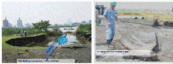
Photo 1 Leakage accident at a distribution pipe (inner diameter: 1,500 mm)
