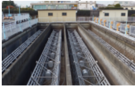
Fig. 8 Floculators in the flocculation basin (Flame type)
