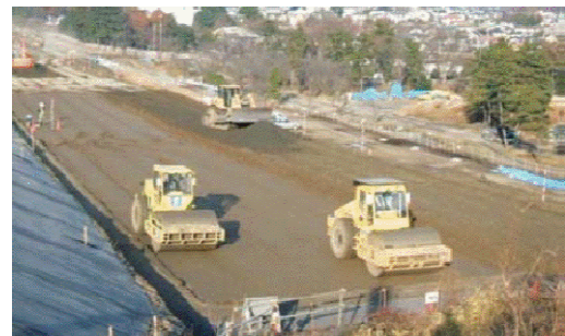
Fig. 9: Reinforcing embankment materials Levelling and compaction
