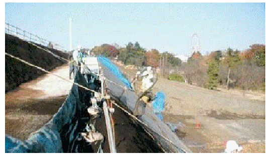
Fig. 11: Downstream slope preservation work (spraying thickening material)
