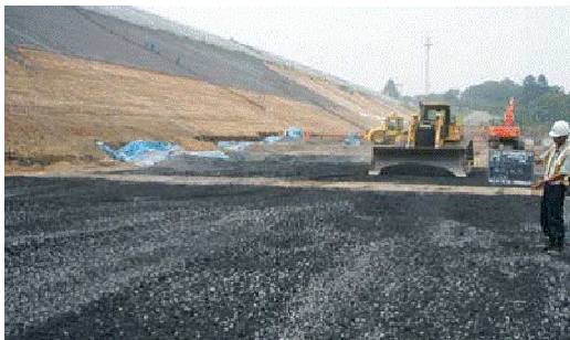
Fig. 8: Horizontal drain Levelling and compaction
