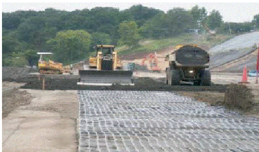
Fig. 10: Geotextiles Reinforced soil embankment fill
