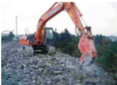
Fig. 6: Bomb-protection layer removal
