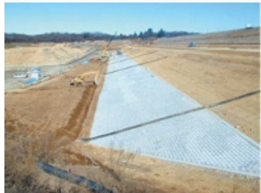
Fig. 4: Concrete blocks (Upstream side)
