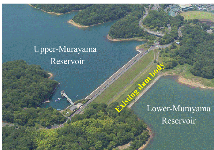
Fig. 13: Upper-Murayama Reservoir Dam Body after an earthquake directly beneath the city of Tachikawa, after which the top of the reinforced dam body would settle by 53 cm. This satisfies the target evaluation standard of settlement under 1.0 m.
