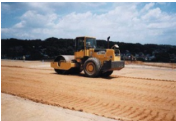
Fig. 3: Compaction
