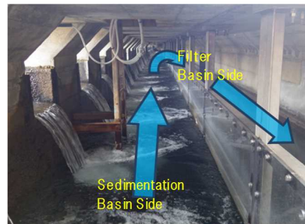
Figure 17 Partition wall installed in sedimentation water channel
