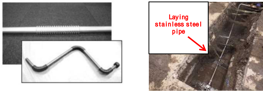
Figure 8 Stainless Steel Pipes (Water Service Pipes)
