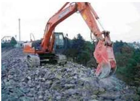
**Fig. 6:** Bomb-protection layer removal
