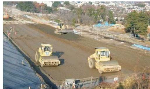
**Fig. 9:** Reinforcing embankment materials
