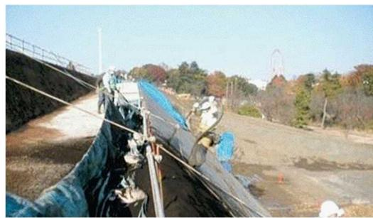
**Fig. 11:** Downstream slope preservation work
