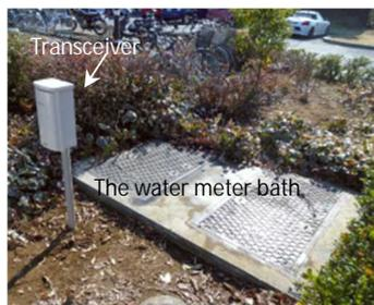
**Figure 9** Transceiver installation (Facilities A and B)
