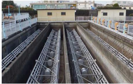
**Fig. 8 Flocculators in the flocculation basin (Flame type)**
