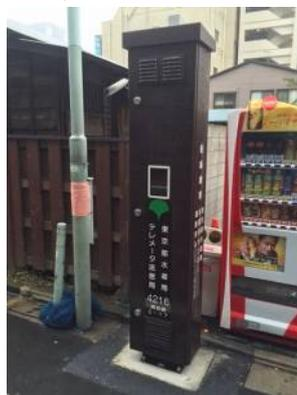
Figure 7 - Thin-type telemeter
