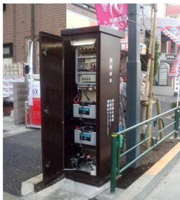
Figure 6 - Aboveground telemeter equipped with rechargeable batteries
