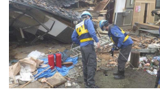
Figure 2. Emergency restoration activities after the Kumamoto Earthquake
