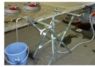
Fig. 3: Emergency water supply from a fire hydrant
