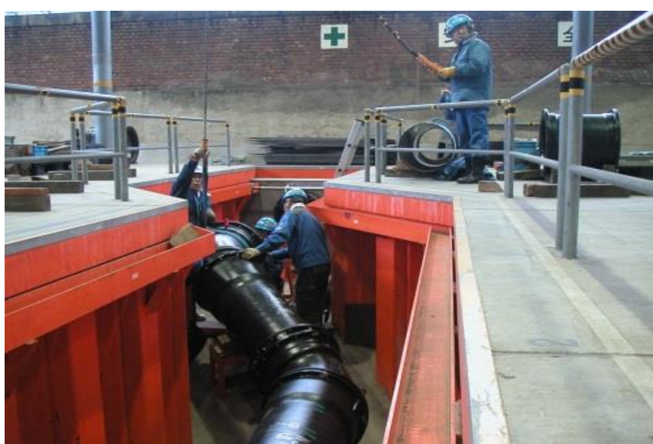
Figure 2: Large-diameter piping practice facility
