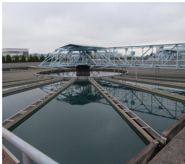
Liyutan Purification plant
