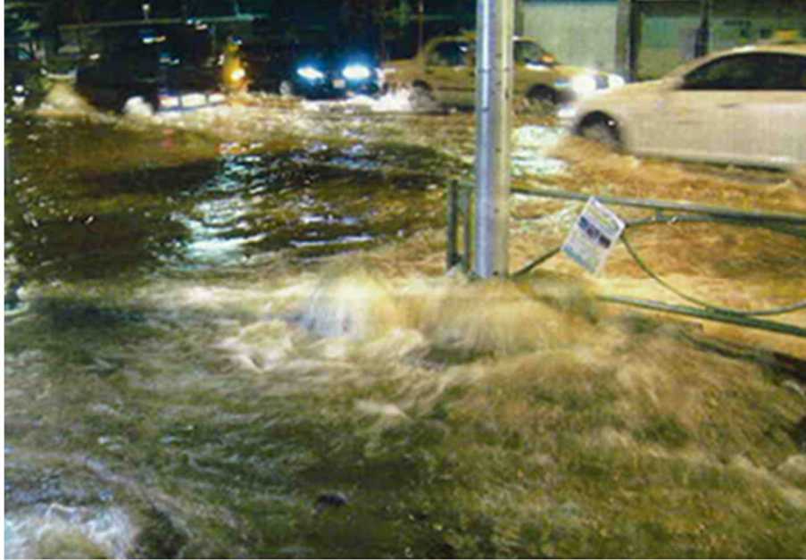
Fig.4-1 Scene of leakage
