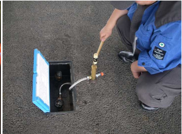
Fig.24 Water hammer Generator
