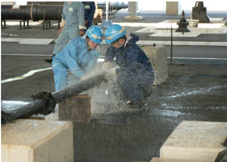
Fig.13 Technical training for leakage prevention work
