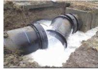
Figure 2: Slipping off of large diameter pipes (Source: MHLW)
