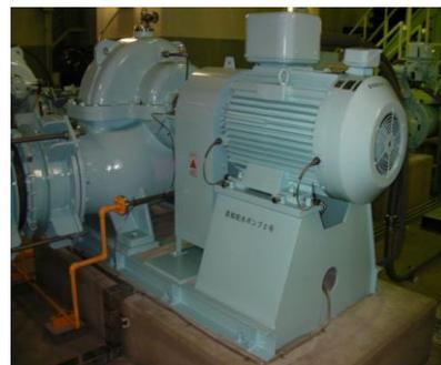
Figure 15 Sample installation of directly-connected water distribution pump
