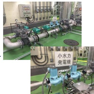
**Figure 11** Serial connection of hydraulic generators
