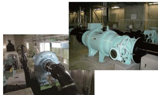
Figure13 Hydraulic power generation Equipment at water supply station
