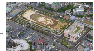
Completed Kouemon Water Supply Station
